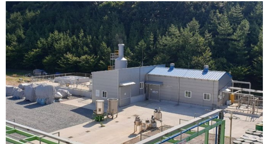
Wastewater treatment facility
