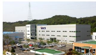
Daesan Plant (Headquarters)
