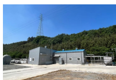
Water treatment facility in Daesan Plant
